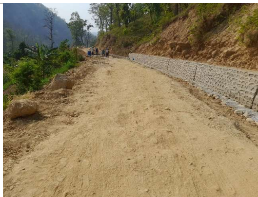
Figure 2 Road upgrading- Bheriganga 5
