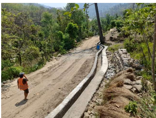
Figure 3 Upgraded road- Bheriganga 4
